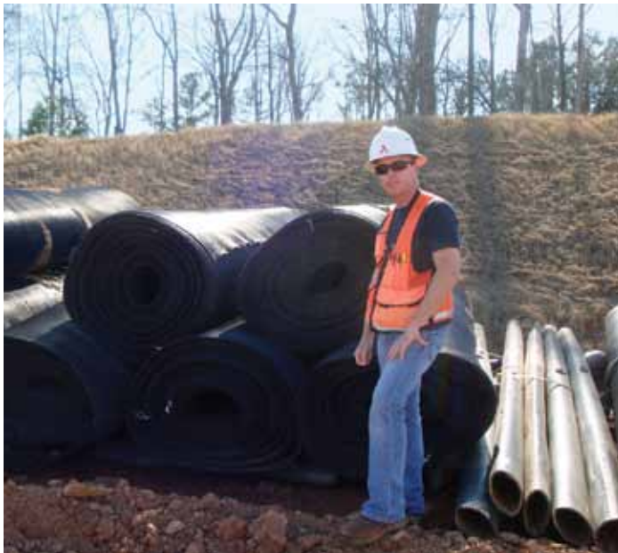
David Duncan, construction leader, alongside liner materials to be used at a gypsum landfill at Plant Wansley in Georgia.
